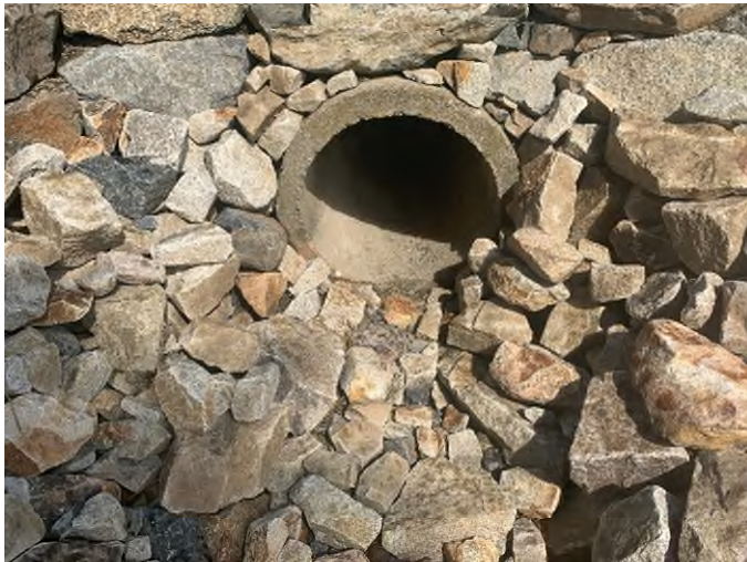
64 Gundalow - 1 (Drainage Course)
