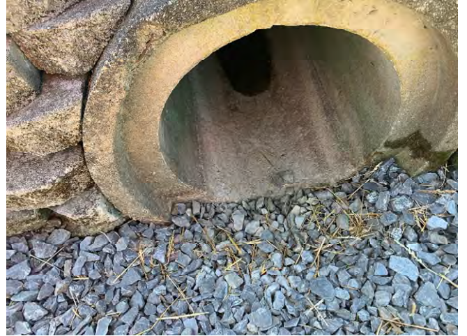
29 Gundalow - 1 (Drainage Area)
