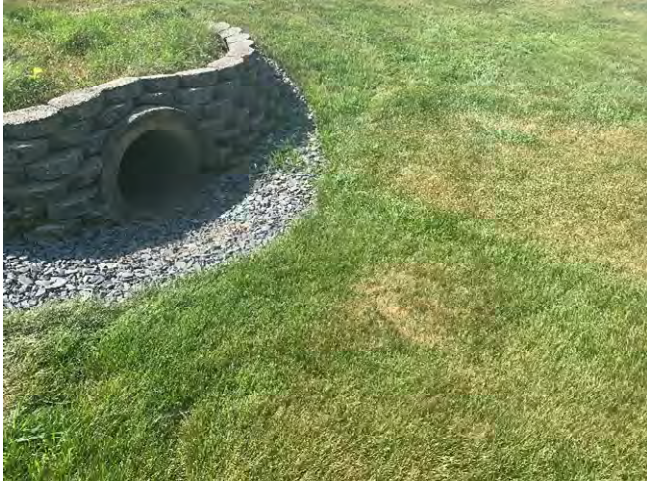
29 Gundalow -1 (Drainage Area)
