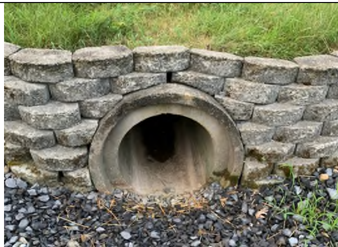
29 Gundalow -1 (Drainage Area)
