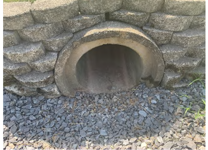
29 Gundalow -1 (Drainage Area)
