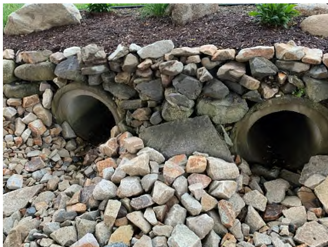
64 Gundalow - 2 (Drainage Course)
