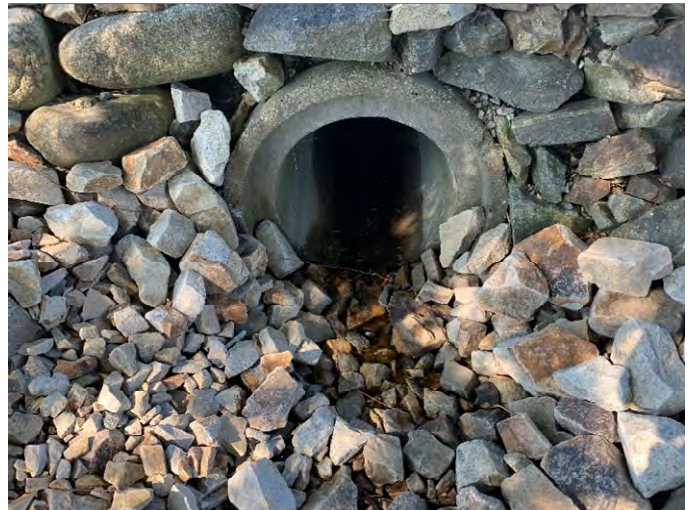
64 Gundalow - 2 (Drainage Course)
