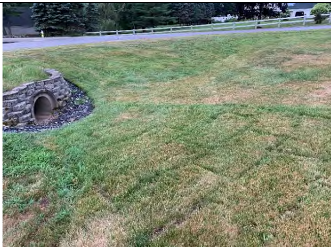
29 Gundalow -1 (Drainage Area)
