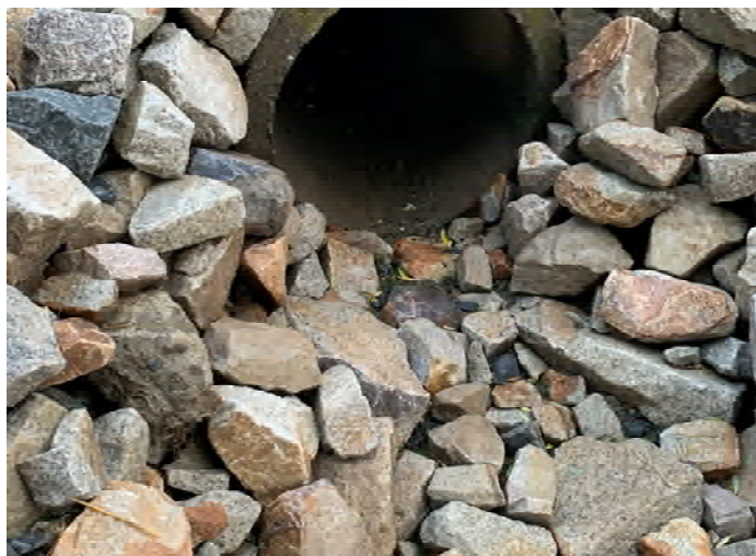
64 Gundalow - 1 (Drainage Course)
