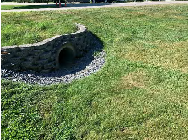
29 Gundalow - 1 (Drainage Area)
