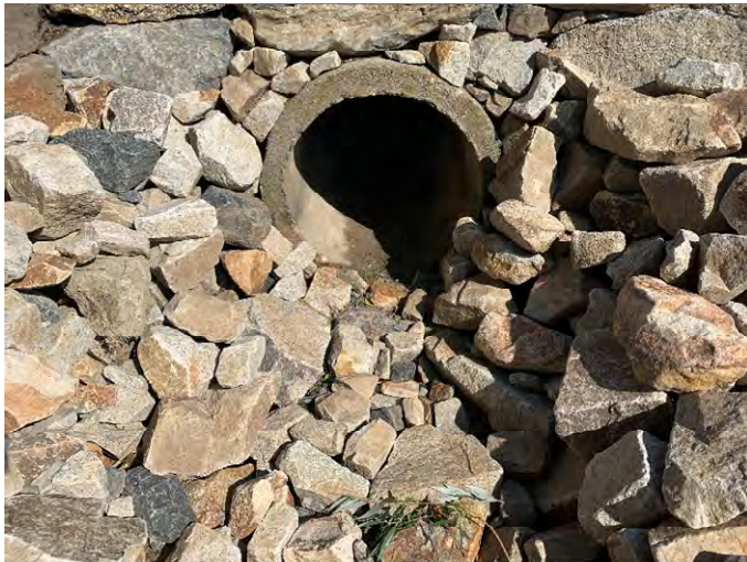
64 Gundalow - 1 (Drainage Course)
